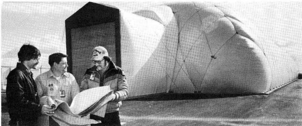
BLOWN out of all proportion? No indeed, it is Sandia's largest inflatable building located just south of Area IV. It is 60 ft. wide by 200 feet long and contains 500,000 cubic feet of storage space. Being totally air-supported, the balloon building has no internal support structure. It's be-
